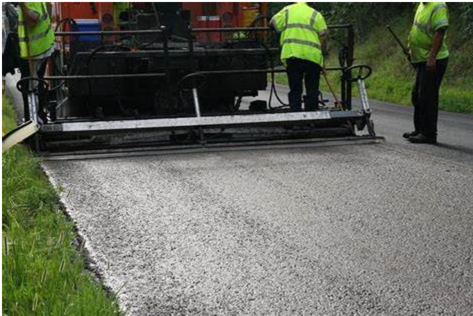
Figure 18: Typical Microsurfacing Paving Crew
